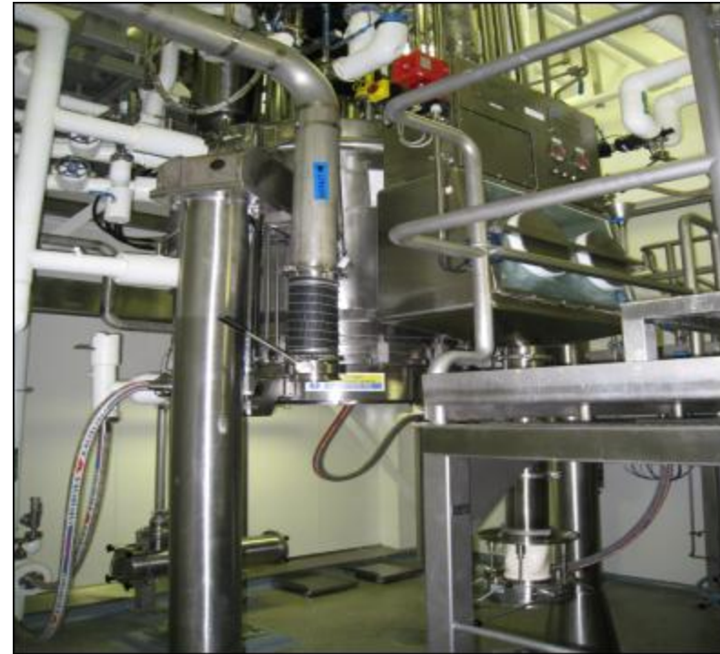
Filter dryer with discharge arm located under glove box
